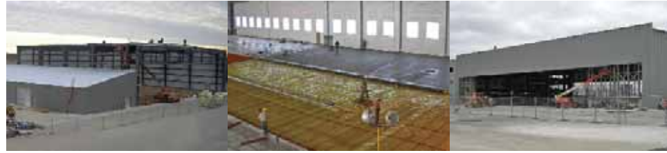
(below L to R) The roof of the new paint hangar is put in place; the new hangar floor is installed; the doors of the new hangar are installed. (opposite page) Steel framing on the new maintenance hangar.
