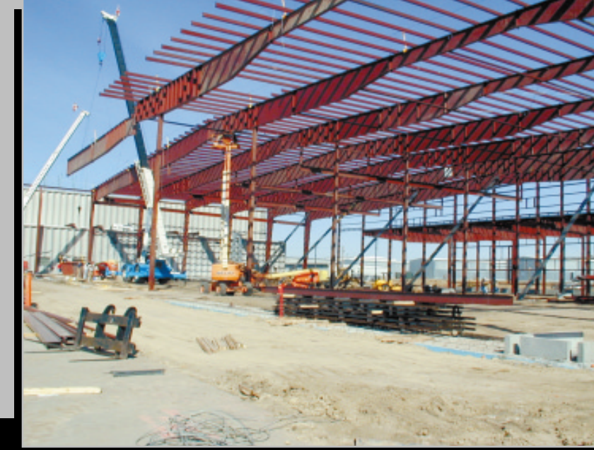
Steel for the hangar and shop space structures began arriving in early January 2000. The metal weighs 2,818,000 pounds (1,406 tons) and was delivered in 75 truckloads. (Left and Bottom)
