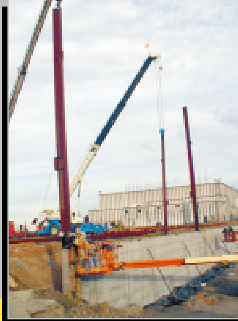
Steel for the hangar and shop space structures began arriving in early January 2000. The metal weighs 2,818,000 pounds (1,406 tons) and was delivered in 75 truckloads. (Left and Bottom)
