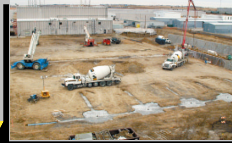
The hangar foundation and the basement area walls were poured in early December 1999. They contain 296,363 pounds of reinforcing steel and 19,440,000 pounds (9,720 tons) of concrete. (Right)
